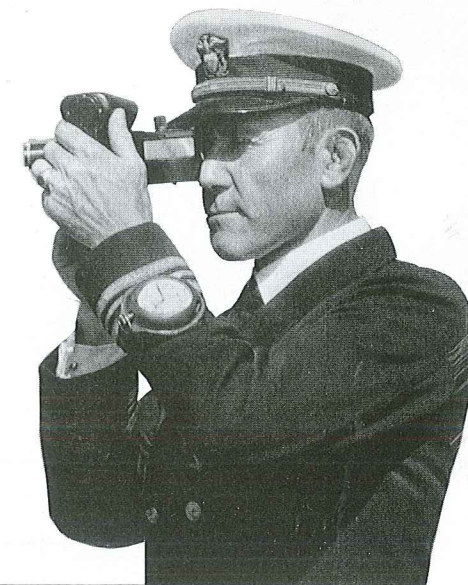
Lt. Commander Philip Weems demonstrating a modified sextant, which could be used independently of a visible horizon. Weems is wearing his second-setting watch on his left arm.
